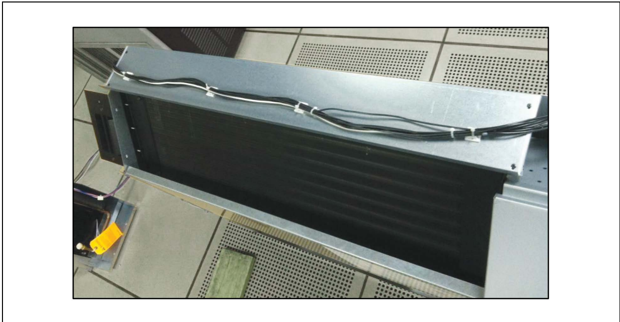
Figure 4.12 Power/Control Wire Harness Routing
