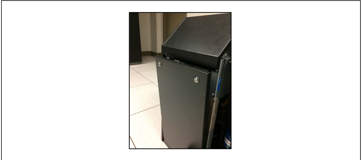
Figure 4.7 Remove Front Access Panel from Condensing Unit
