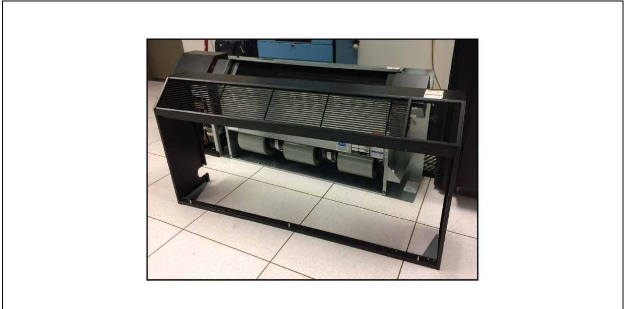
Figure 4.3 Remove Evaporator Panel Assembly
