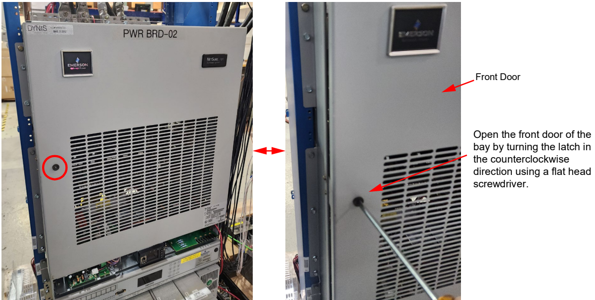
Figure 2.3 Opening of the Front Door
