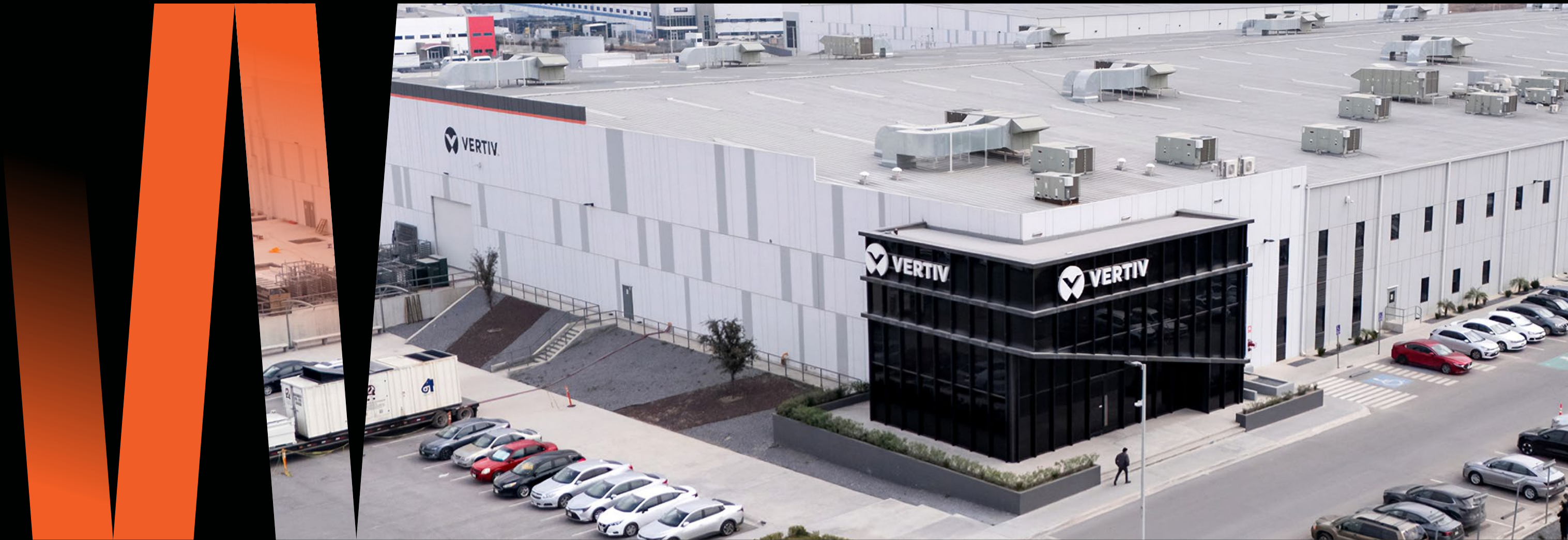
Vertiv manufacturing facility, Monterrey, Mexico
