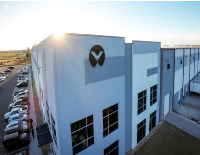
Vertiv manufacturing facility, Pelzer, South Carolina, USA
