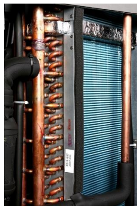
Figure 1-4 Cooling coil
