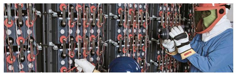
Frequent internal resistance testing helps you understand the health of your batteries and ensure network reliability.
