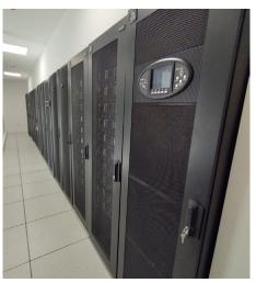
The engineering of Nini's new data center was no small task. For starters, the Vertiv team had to ensure the technical floor would support the weight of the Liebert® APM unit that was to be enclosed in a protective rack. Following weight calculation, structural modification ensured the floor could handle the 1,200-kilogram solution.
